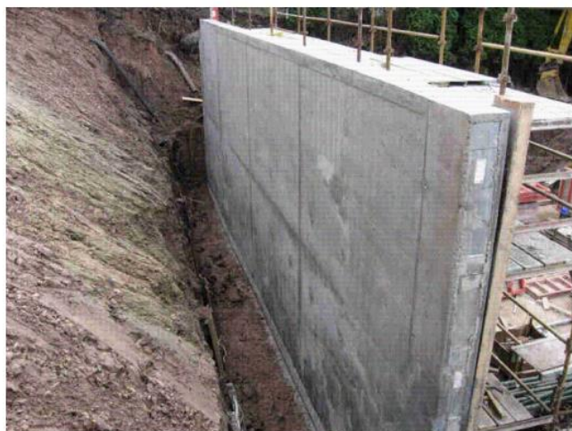
Figure 14: Typical batter back excavation and RC retaining wall construction
