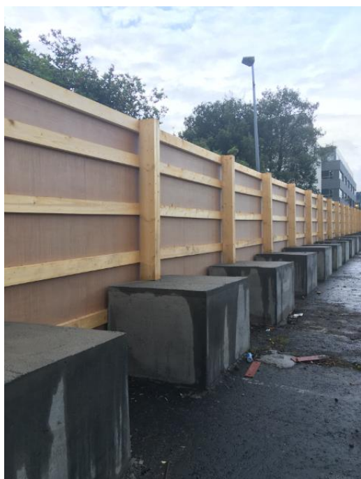
Figure 6: Site hoarding along the eastern boundary
