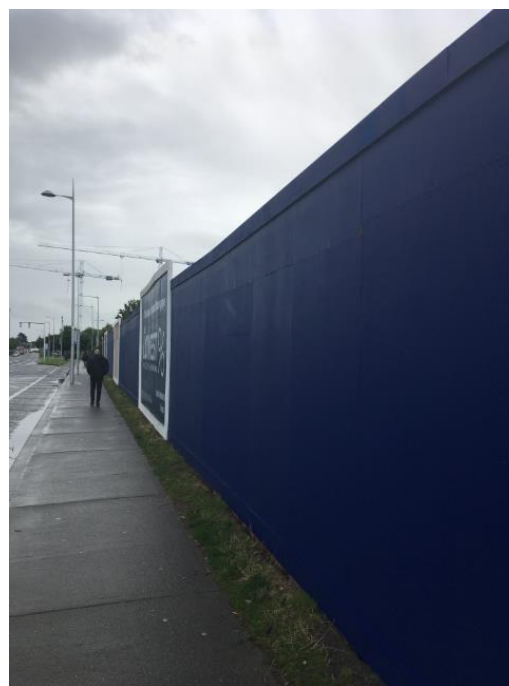
Figure 7: Site hoarding along Blackthorn Drive
